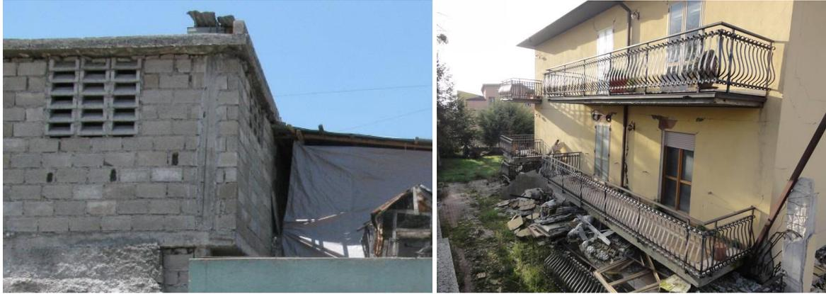
*Figure 9: Vulnerability Modifiers: Poor quality confined masonry construction, Haiti, EEFIT, 2011 (left); irregularities in plan i.e. soft storey, L'Aquila, 2009, EEFIT (right). Poor quality construction and irregularities in the plan, both increase a building's vulnerability thus a higher vulnerability class will be assigned by identifying these features from the photograph.*
