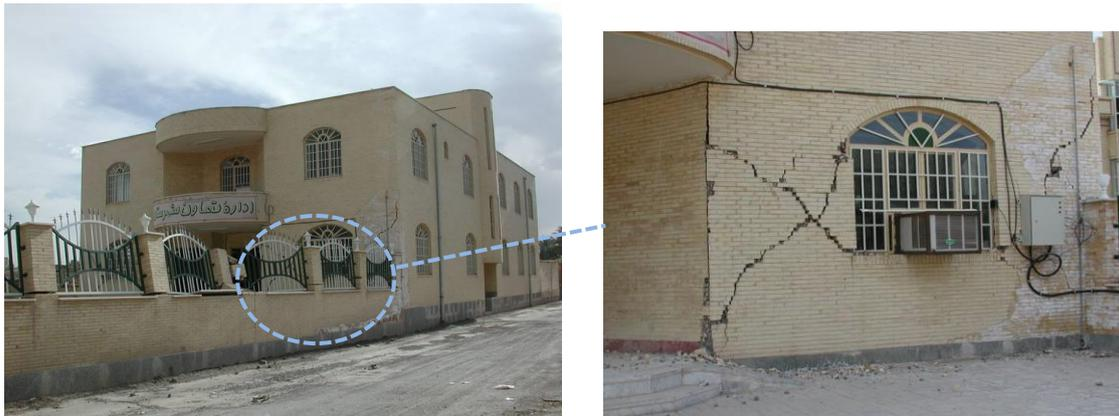
Figure 7: Overall structure (left) and detailed photograph (right) of a reinforced concrete frame building with brick infill walls, Bam, Iran, 2003. Source: EERI. A "detailed photograph" (right) provides a remote analyst with additional detail regarding the material type and damage to the building.
