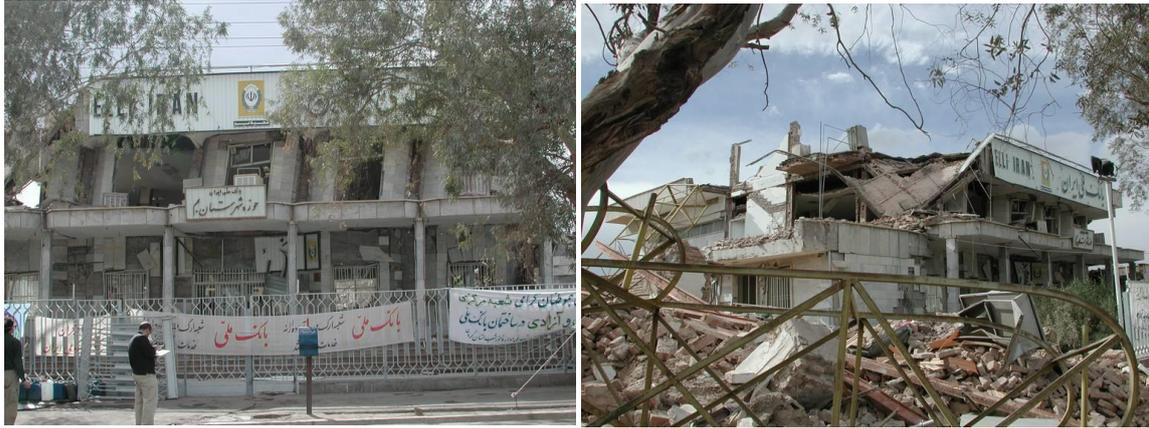
Figure 6: Front (left) and side (right) elevation of a reinforced concrete frame building, Bam, Iran, 2003. Source: EERI. It is vital to have pictures of a range of elevations to understand the entire structural system and assign accurate damage levels i.e. if only one photograph was supplied, the front elevation would be assigned damage level D3, whereas the side elevation would be assigned D4.
